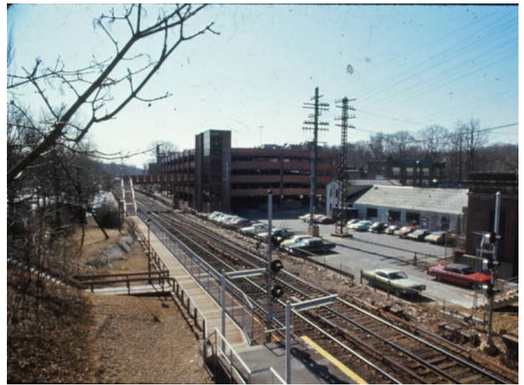
Freightway Parking Garage - 1978
