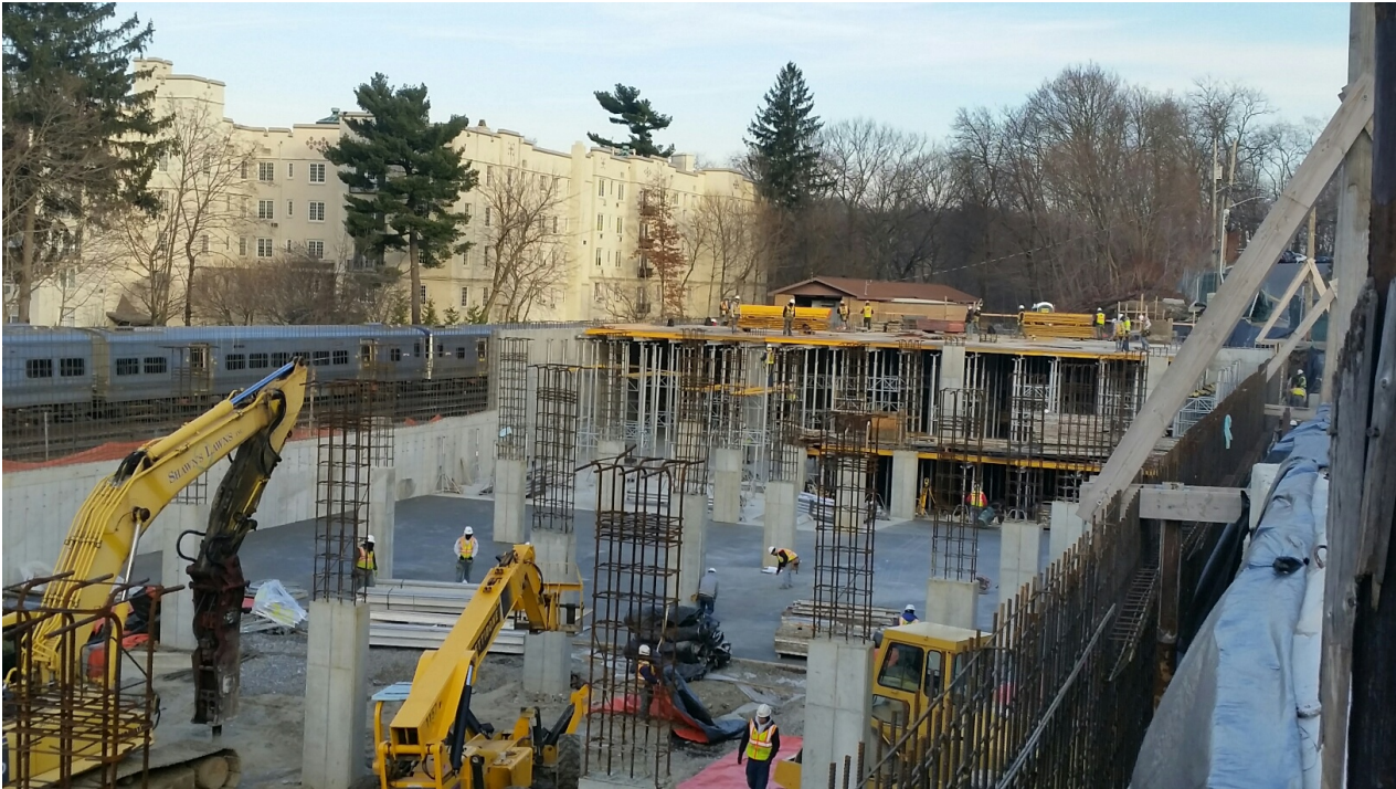
VillaBXV and Parking Garage Construction Adjacent to Metro North Train
