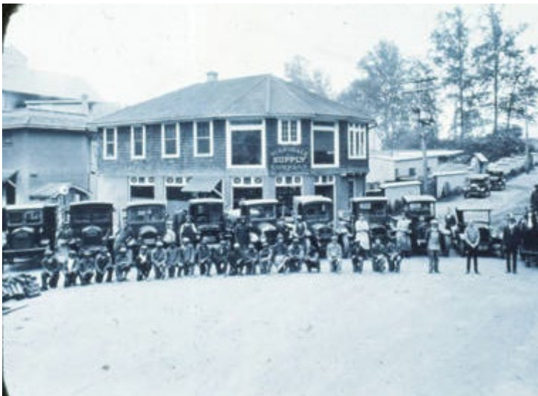
Scarsdale Supply Company on the corner of Garth and Freightway - 1927
