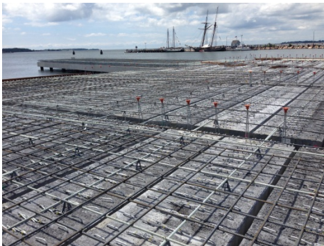
Platform under construction
