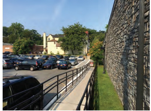
Freightway site connection to the southbound Metro-North platform via the Popham Road Bridge
