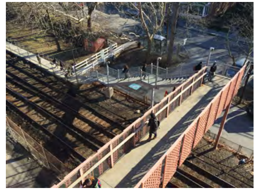
Pedestrian Bridge to Scarsdale Avenue
