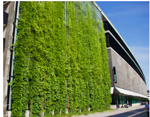
Cable supported green wall in Switzerland
