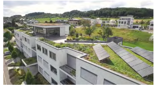
Green roof with solar panels
